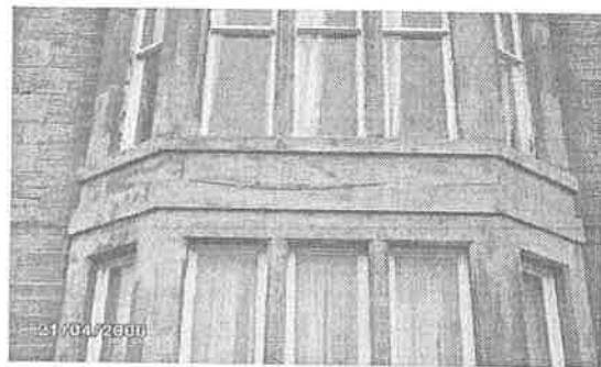
Figure 6. Sandblasted bay window
