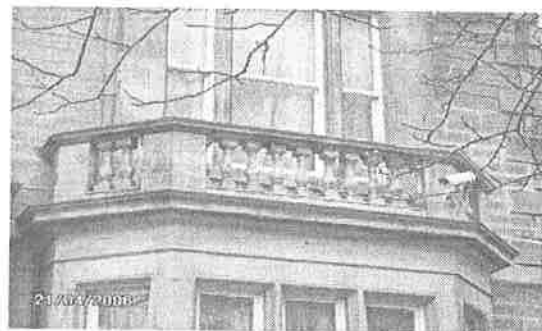
Figure 8. Sandblasted front balcony
